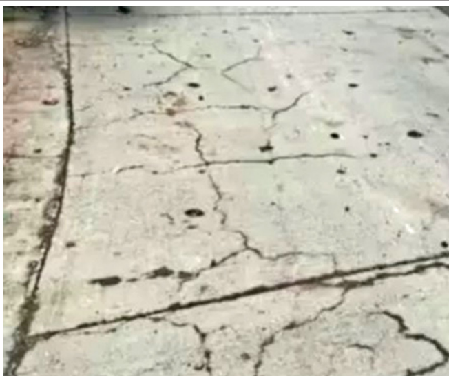
Fig. 10. Cement concrete pavement with visible cracks allowing percolation of rainwater at IIT Roorkee.
