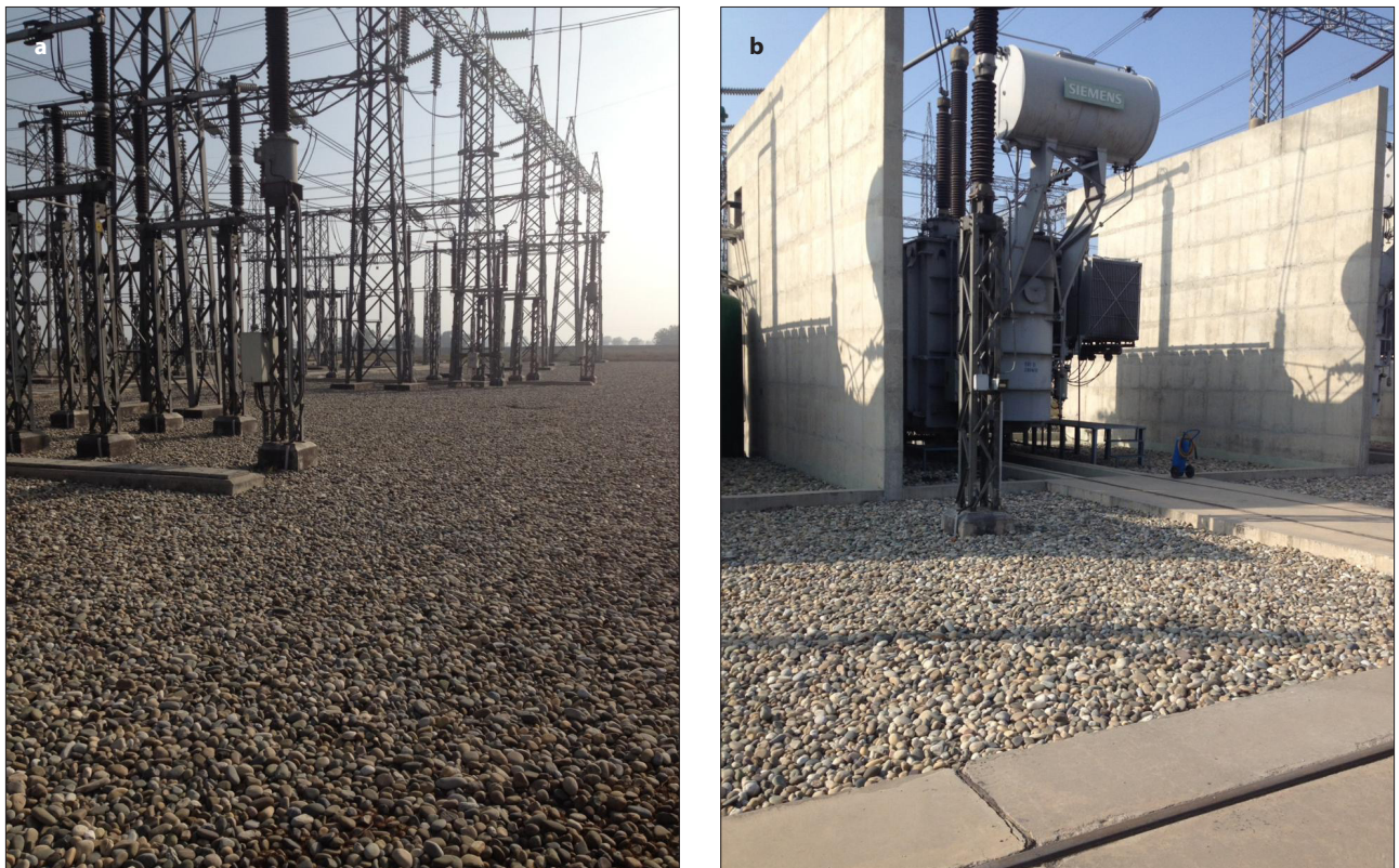
Figure 1. a, b. Photograph of NOKHAR substation showing gravel as surface material in the switchyard (a). Photograph of NOKHAR substation showing concrete as surface material on the pathways (b)
